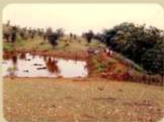
Drainage line treatment
