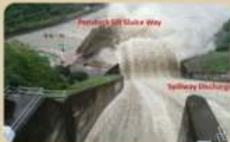
Simultaneous operation of spillway and penstock sluice venting turbid density current
